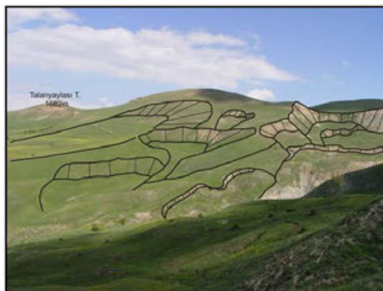
Figure-6. A general view of wide spread landslides developed from 1 km NE of Dumlusu towards SW (J47 d4, 20 500-22 750, looking North).
