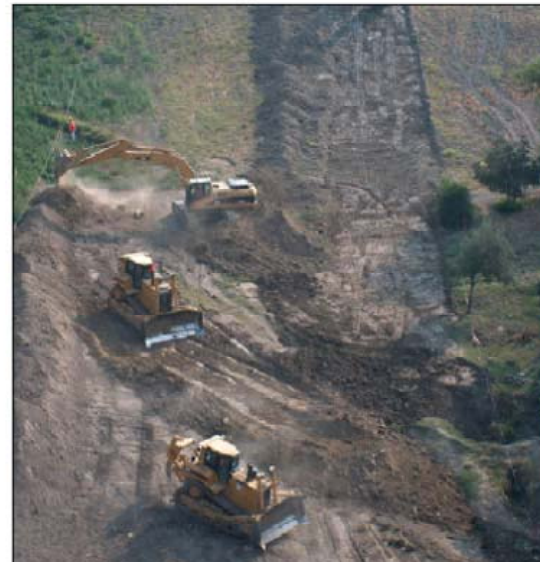
TOPSOIL STRIPPING
