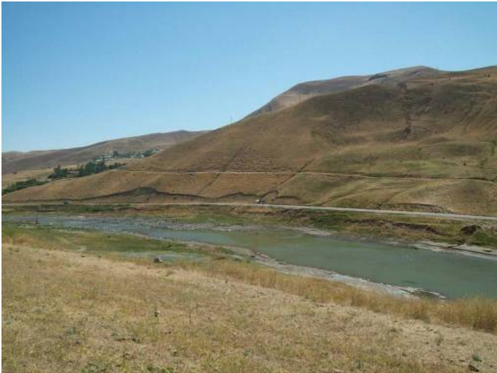
Photo 5: Opposite bank of the construction site of the main body of the ALP-D-HEPP
