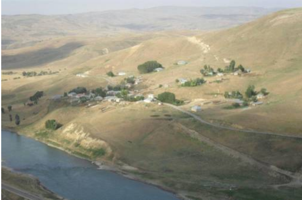
Photo 6: Construction site for the inlet of the derivation tunnel of the ALP-D-HEPP
