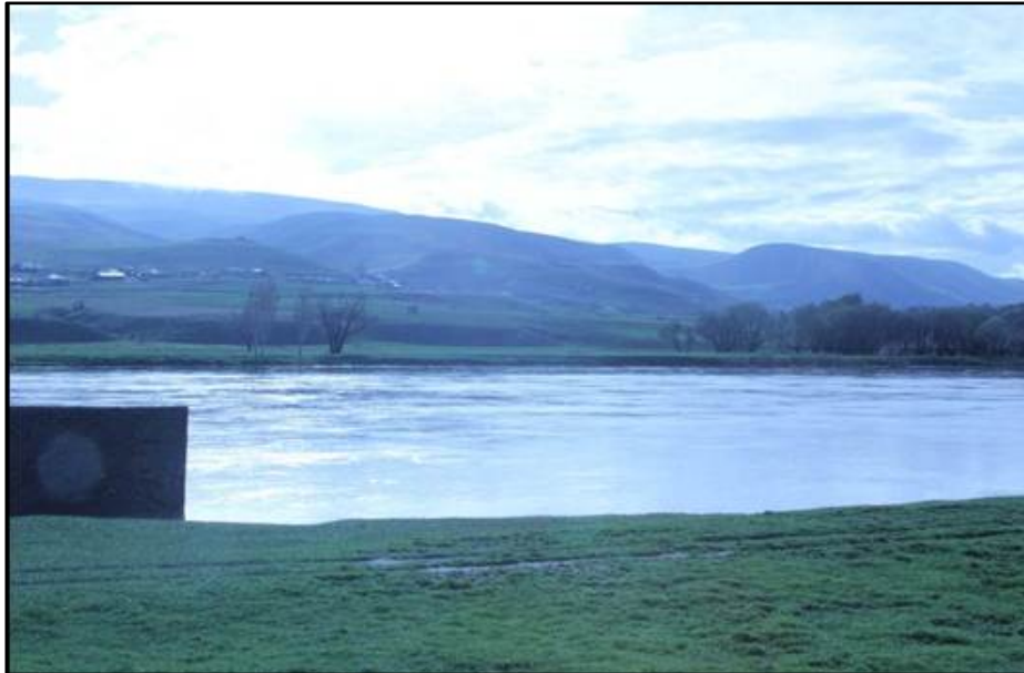
Figure C.1. General View of Alpaslan II Dam Typical Riverbed
