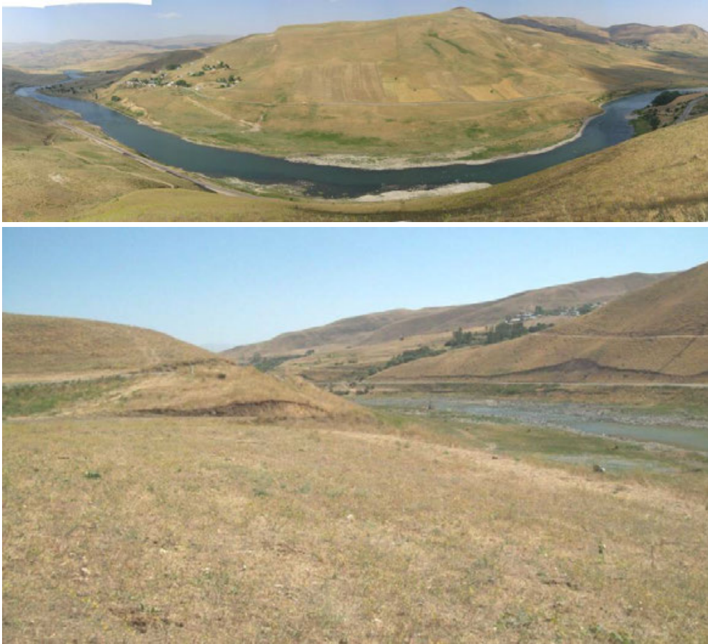
Photo 4: Construction site of the main body of the ALP-D-HEPP
