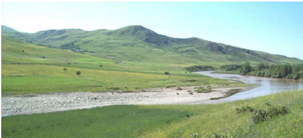
Photo 9b: Riverbed excavation sites for providing permeable materials (sand)
