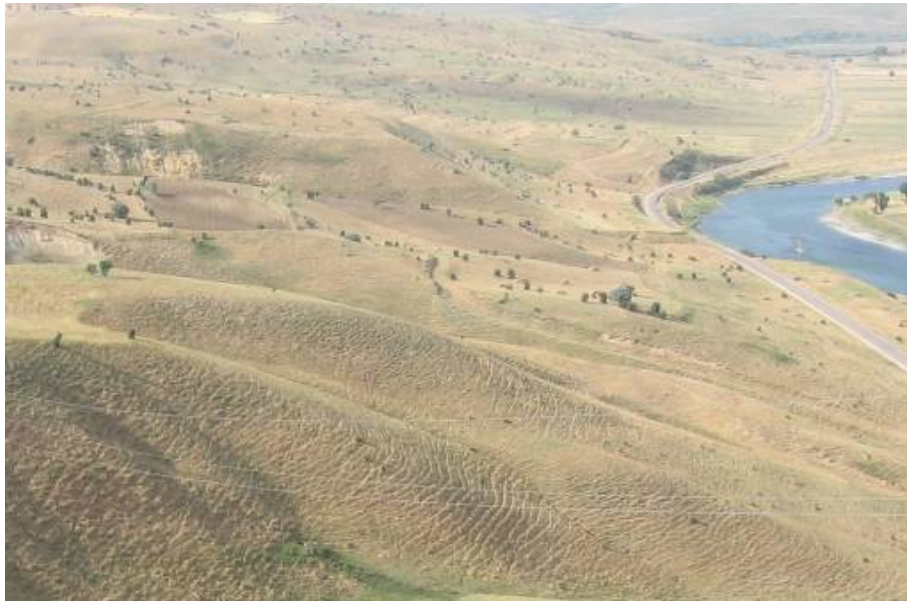
Photo 8a: The storage area-I of the ALP-D-HEPP
