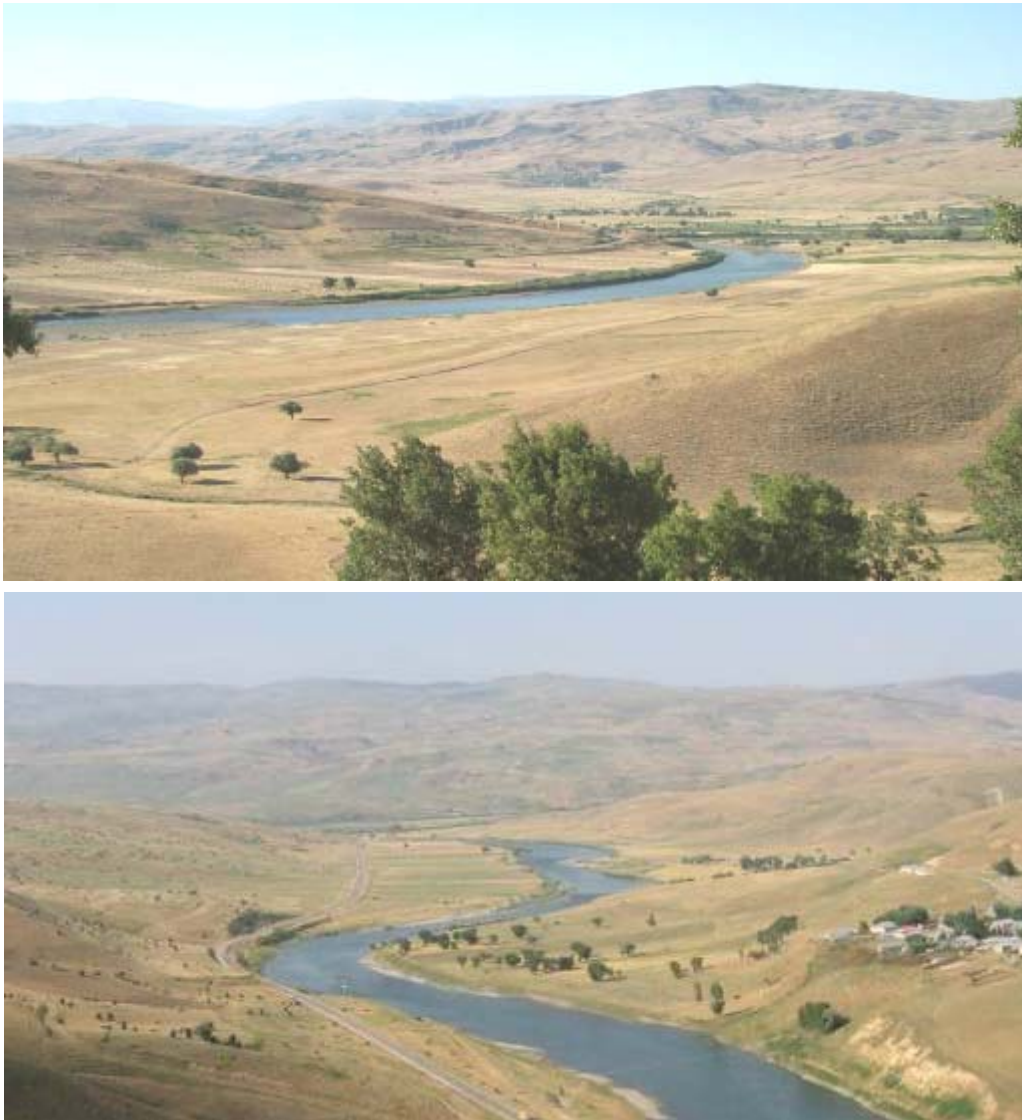
Photo 8b: The storage area-II of the ALP-D-HEPP
